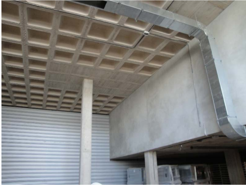
VISTA INTERIOR GARAJE
